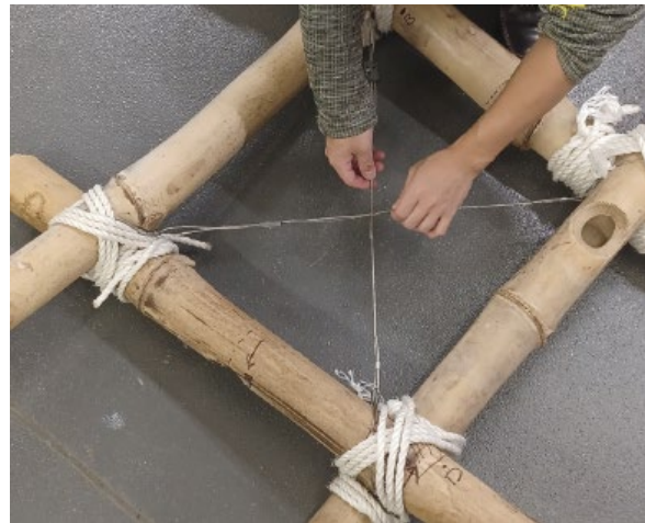
Figure 6 Tensioning and lashing a reciprocal unit
